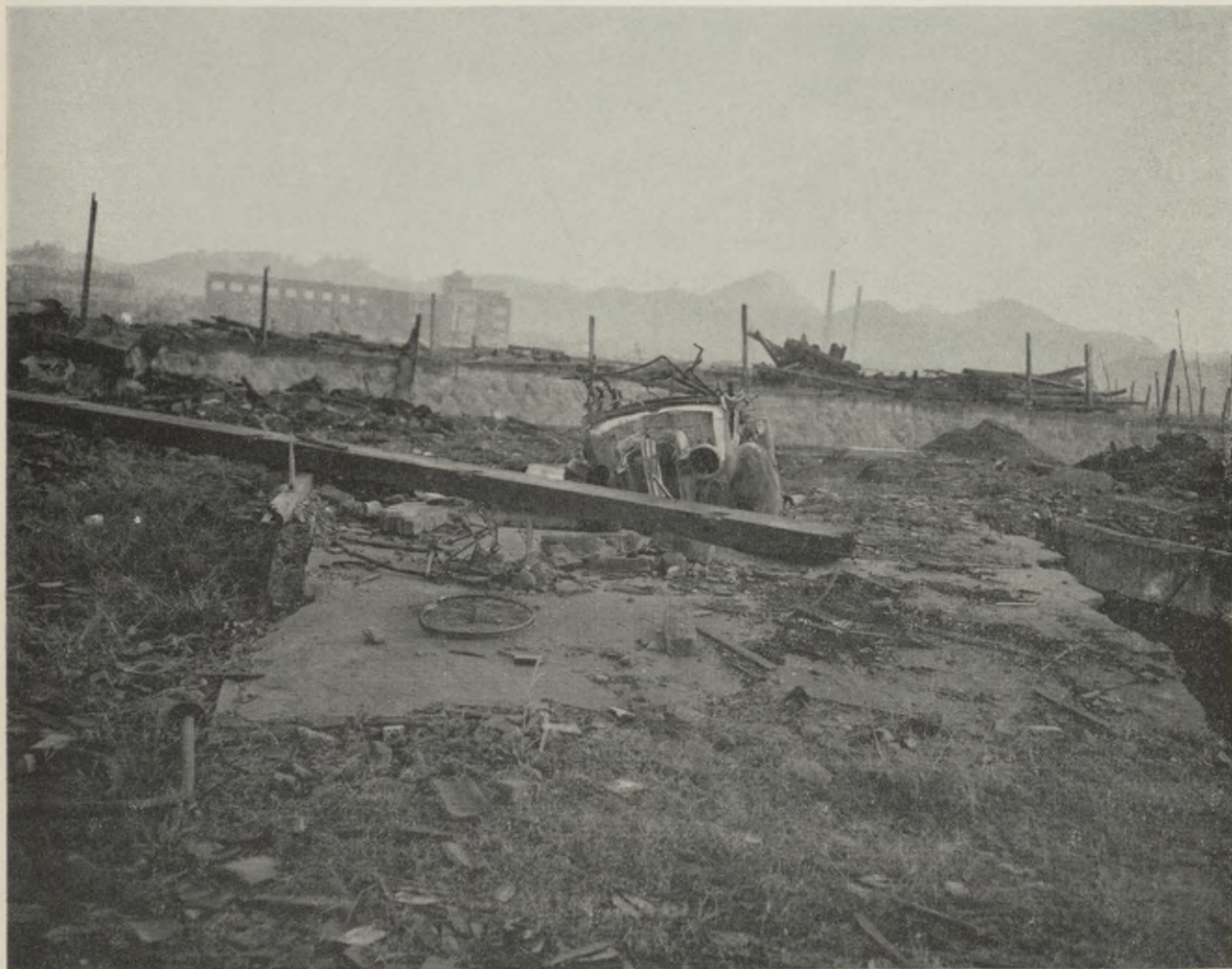
Photo 14. Ohashi Substation, completely damaged by atomic bomb. Nine firemen, the entire complement of this station, were killed.
